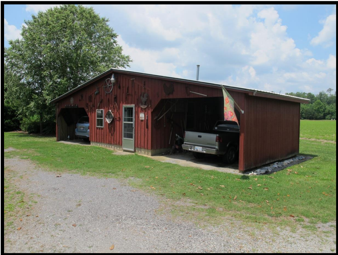
Figure 12: Overflow Farm (# 1), Outbuilding, Looking West.
