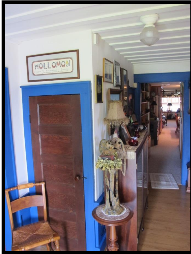
Figure 7: Overflow Farm (# 1), Interior, Center Passage, Looking West.
