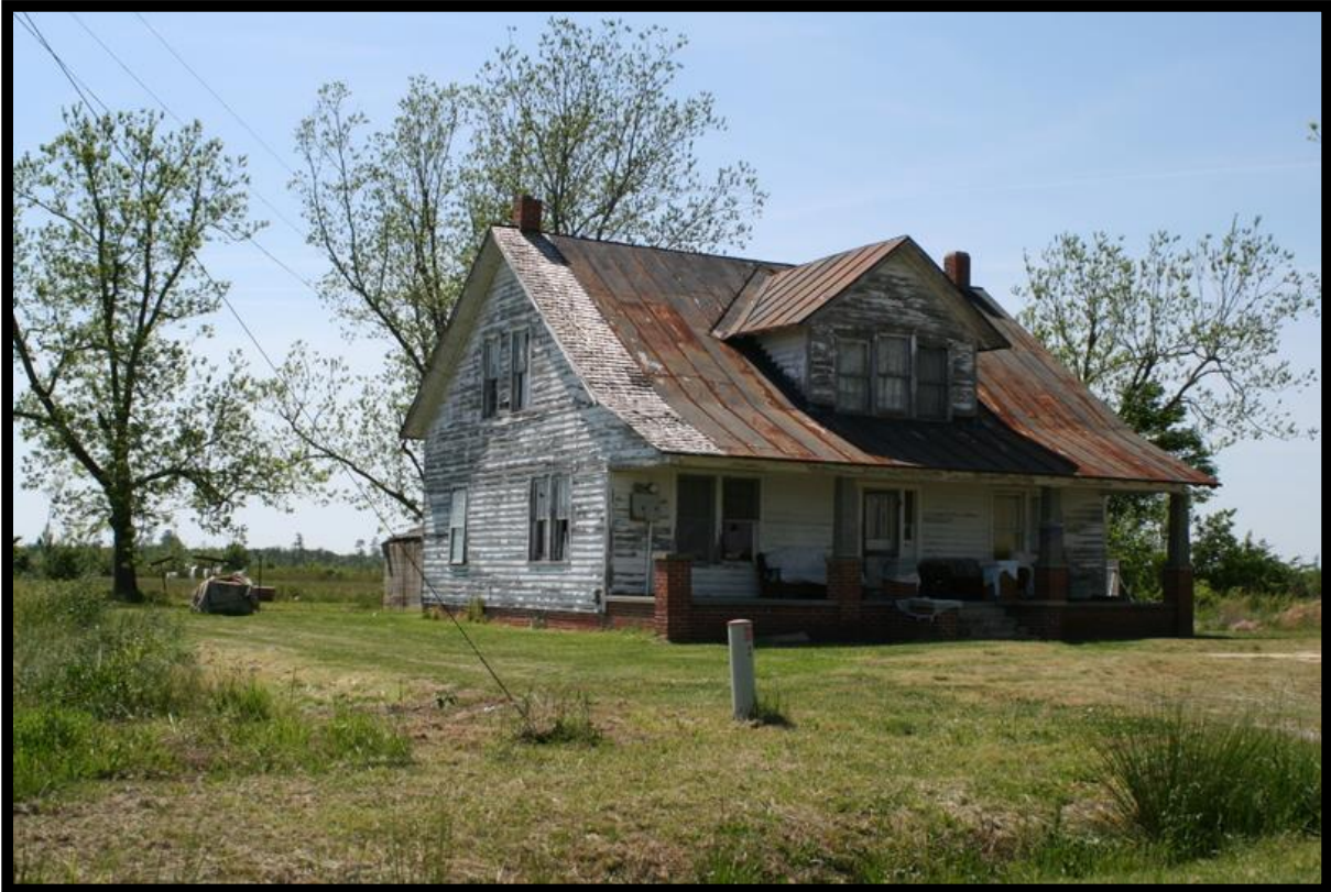
Figure 28: Mitchell House III (BR0618), Morris Farm Road (SR 1342).
